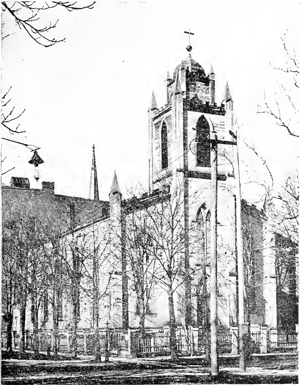
THE OLD ST. MARY'S CHURCH.—From a recent photograph.
